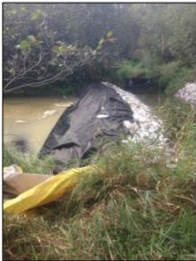
Photos 29-30: Placement of the rock on the berm and opposing shoreline.
