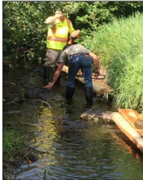
Photos 13-16: Building and installing of ½ logs
