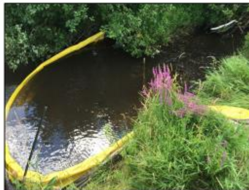
Photo 12: Silt curtain placed in creek to prevent siltation
