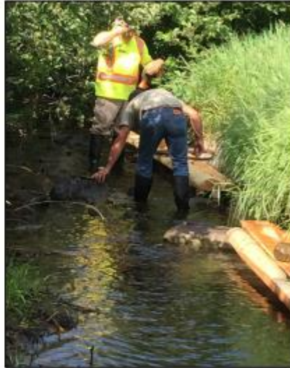
Photos 13-16: Building and installing of ½ logs
