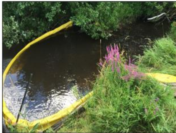
Photo 12: Silt curtain placed in creek to prevent siltation
