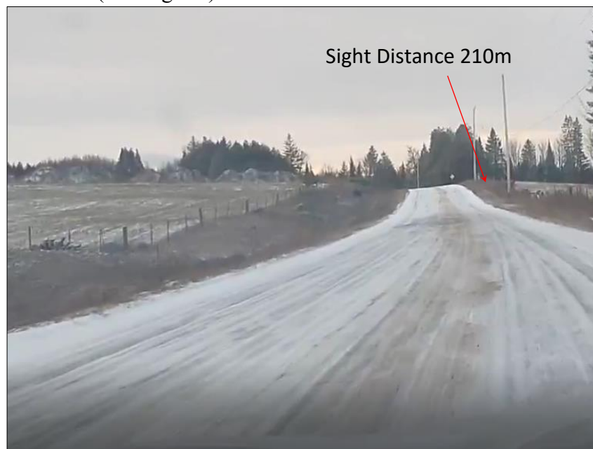
Exhibit 5-11: Alternative Access 1 (EA1) Looking West (210m SD)
